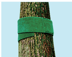
1. Install tree protectors
